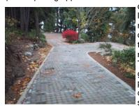
offset by the need for less land, piping and other materials that would otherwise be required for traditional stormwater management practices. The overall maintenance goal for porous pavement/ pavers is to prevent clogging of the void spaces within the surface
